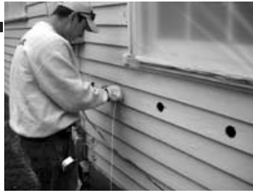
Cellulose insulation is blown into an existing home.
